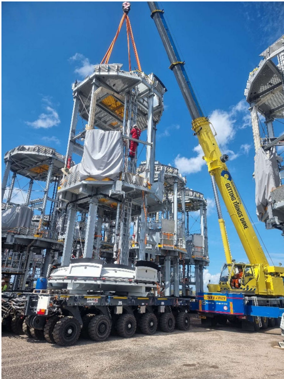
Figure 3, GMK 5130-2 and 6-axle SPMT in action
